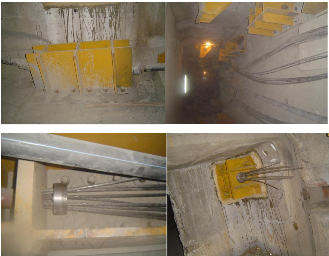
Picture set 1. The steel structures and anchors at the site.
