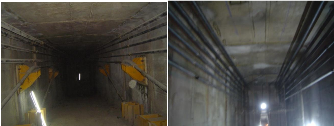
Picture set 3. The span after final external Pre-Stressing by cable bunches.
