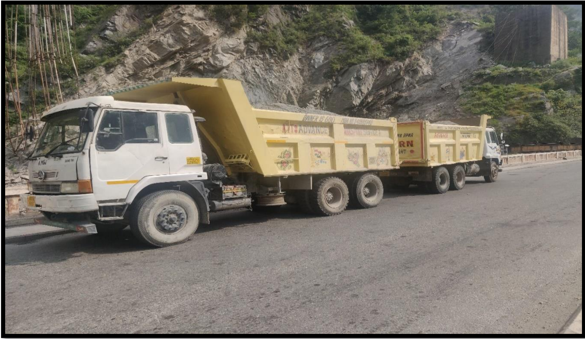
Fig 5 :- Loading arrangements for Static load testing
