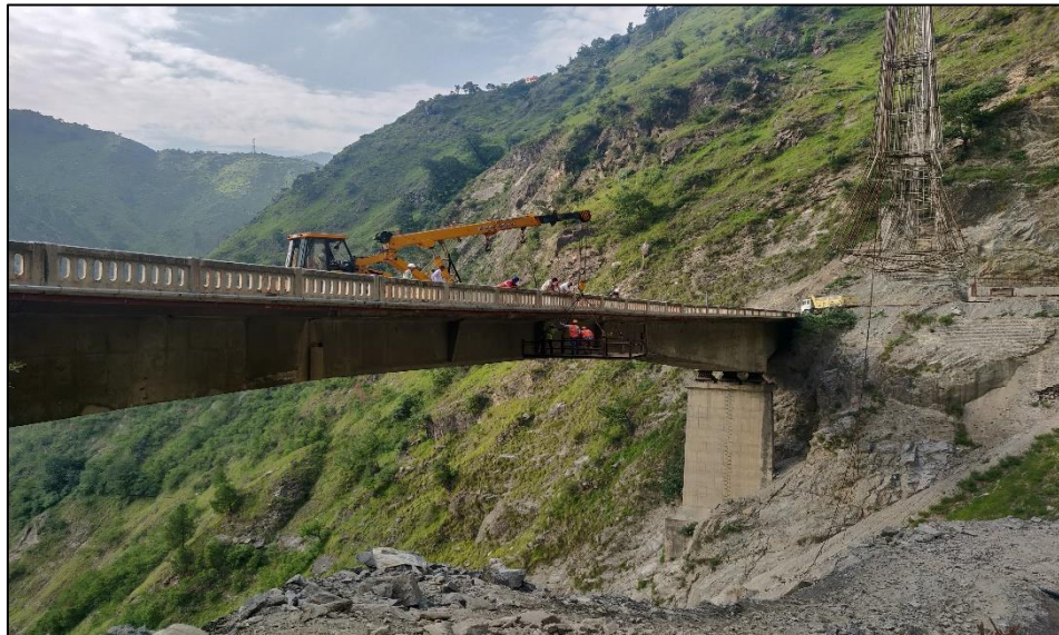
Fig 2:- Crane used to carry out inspection
