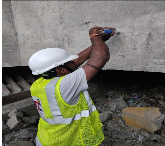
Fig 3: - Rebound Hammer test.
