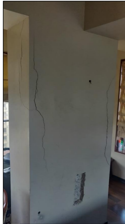
Fig 2: - Major Cracks were detected on Column
