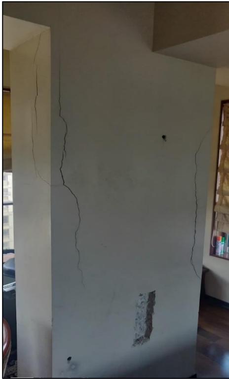
Fig 2: - Major Cracks were detected on Column
