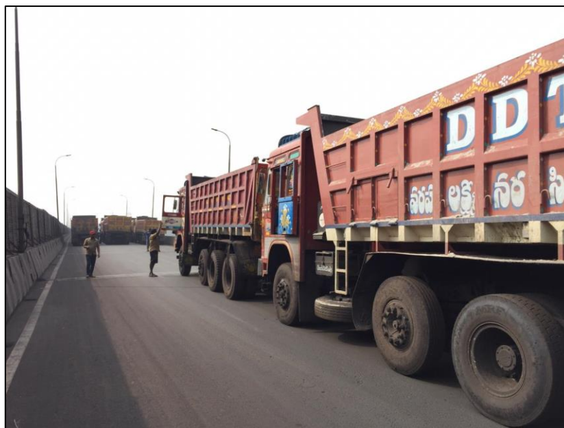
Fig 7 :- Trucks placed for Load testing
