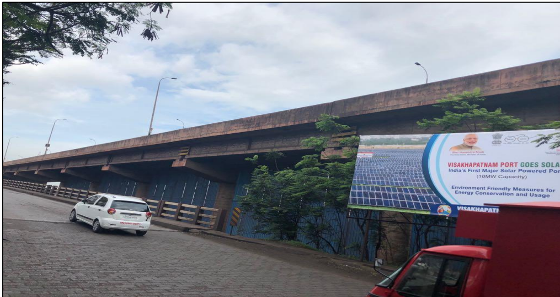
Fig 1:- Visakhapatnam port trust Bridge .
